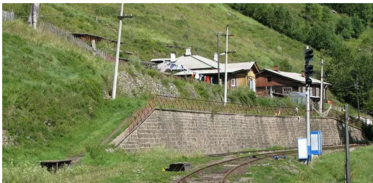
Fig. 9. Granite gneiss blocks. Bridge over the Marituyka River. Photo by the author, 2025.
